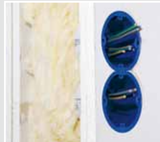
Use of a sound insulation box on one side of a double combination.
