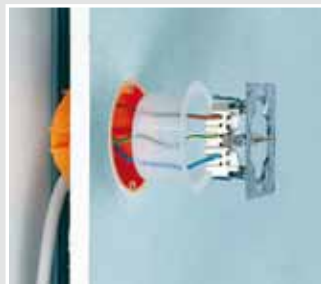
Later air-tight closing of cavity wall boxes.
