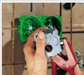
Create a conduit or cable entry (punch pliers or opening cutter).
