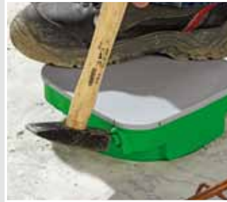
On-site installation: open KSK technology with one blow of the hammer.
