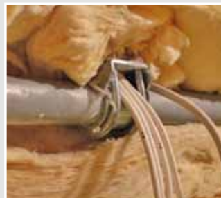
The mast which supports the parabolic mirror must also be incorporated in the equipotential bonding.
