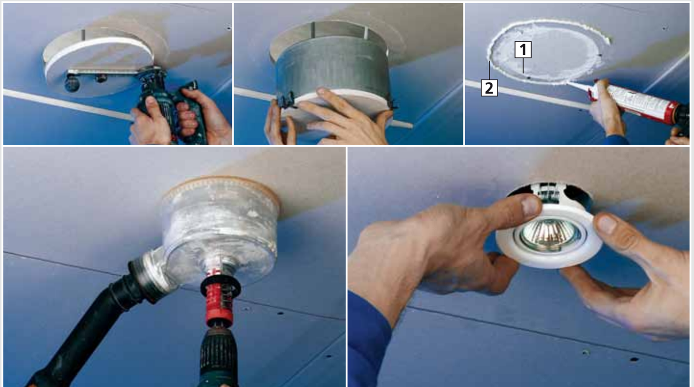
1 Edge joint | 2 Sealing bead
