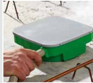
Insert conduits and concrete up.
