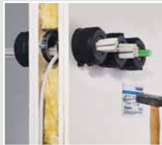
After installing the sealing, apply the identification tag.
