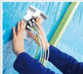
... glue the sleeve in position and thoroughly smooth it onto the surface, working from the inside to the outside.
