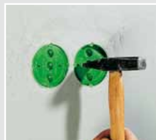
Open concrete building boxes or casings, then fit equipment or cover.
