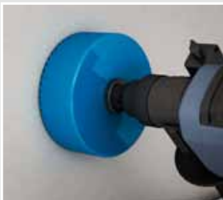
Cut installation opening with a cutter Ø 120 mm (e.g. bi-metal cutter 1082-20).
