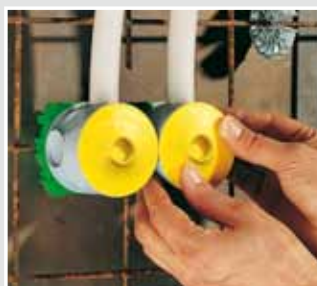
Clip rear part with conduit or cable to front part and concrete.
