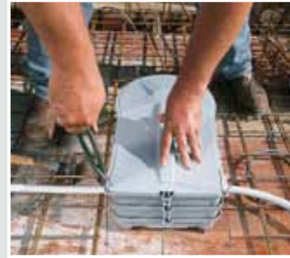
Also secure the housing to the reinforcement.
