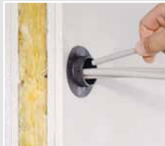
Insert the new cables.
