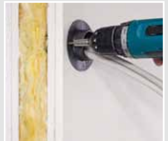
Fasten by tightening the screws (same procedure as for cavity wall boxes).
