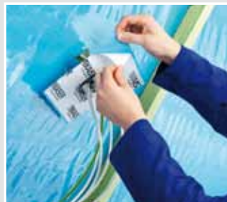
Before the sleeve can be glued in position, make sure that the surface is free of dust. Then remove the protective foil,...
