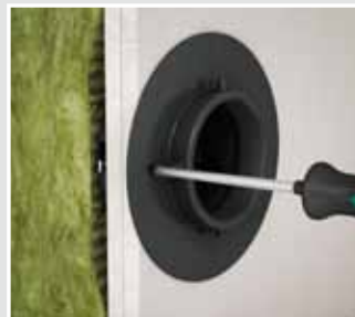
Fix sealing cylinder by tightening the screws (same procedure as with cavity wall boxes).
