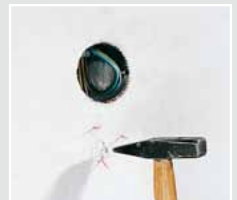
Fine marker bristles on the signal cover show the exact position of the one-gang box after plastering.
