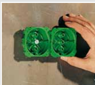
Attach front part to formwork.
