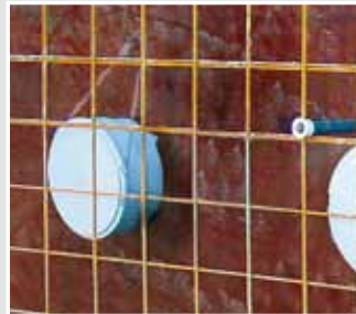
Fasten to the formwork using tensioning wire and nails.
