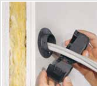
Open the sealing element and remove it.
