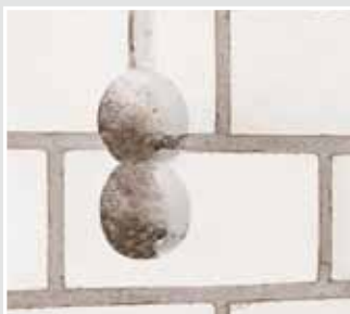
Creating installation opening.
