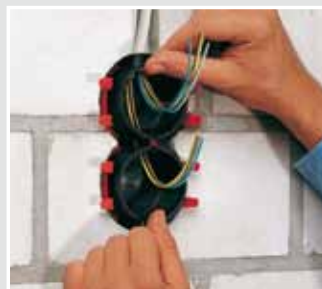
Push in box with Klemmfix® clipped on.
