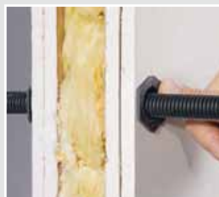
Press both sides of the sealing into each opening.
