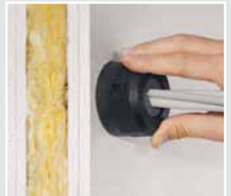
Place the sealing element around the cable, close it and secure it with a 1/4-turn clockwise.
