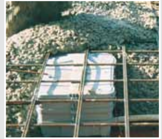
Secure and firm seating of housings during concreting.
