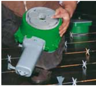
Attach HaloX-P housing with mounting plate to the formwork table using at least 4 pieces of adhesive foil (1219-00).
