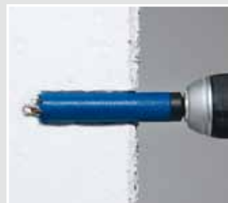
The depth stop ensures that only the amount of insulation needed to secure the mini equipment carrier is removed.
