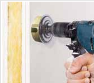
Cut an installation opening using a Ø 74 mm cutter (e.g. Multi 4000: 1084-10).
