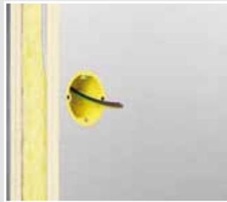
Installation of the radiation protection box in the wall.
