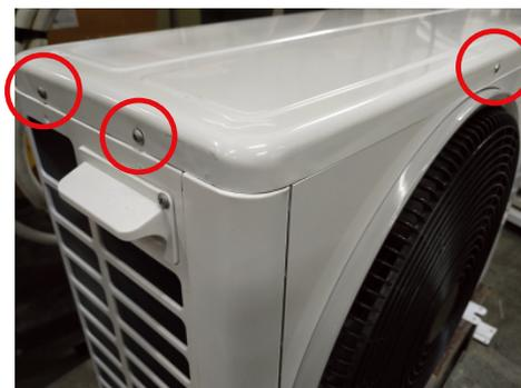
2) Remove the screw fixing Terminal Cover and Cord Clamp, then take them out.
