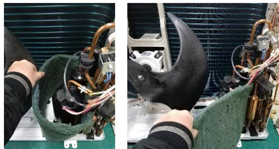
(Disassemble the control box ass'y)
