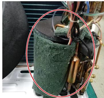
11) Cut the wire fixing band fixing the transfer connector of the compressor and control box ass'y, then disassemble the terminal of reactor and compressor, after all, disassemble control box ass'y.
